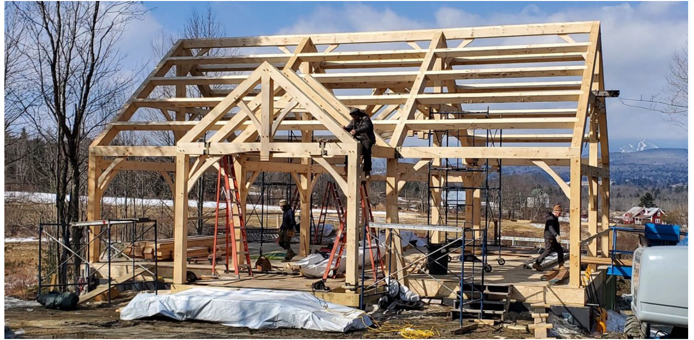
Photo above: Winterwood Timber Frames
